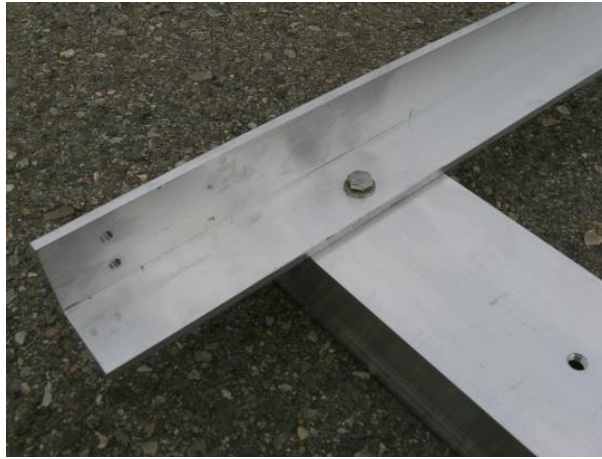
Figure 7 Connection between U- and L-profile
