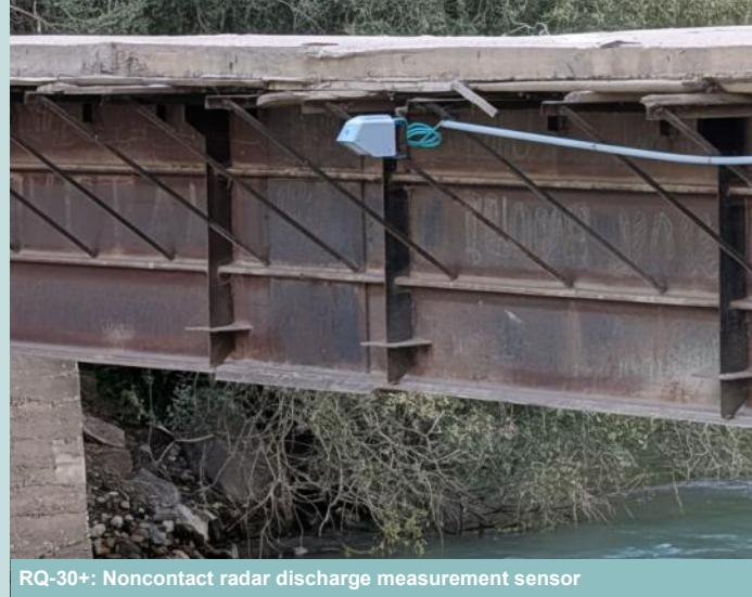
RQ-30+: Noncontact radar discharge measurement sensor
